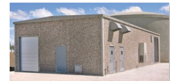
Control Building: Louisiana
