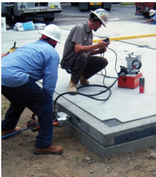
Post-tensioned floor with step-down to ensure weather tightness.
