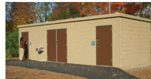
Restrooms and Storage Building: Ohio
