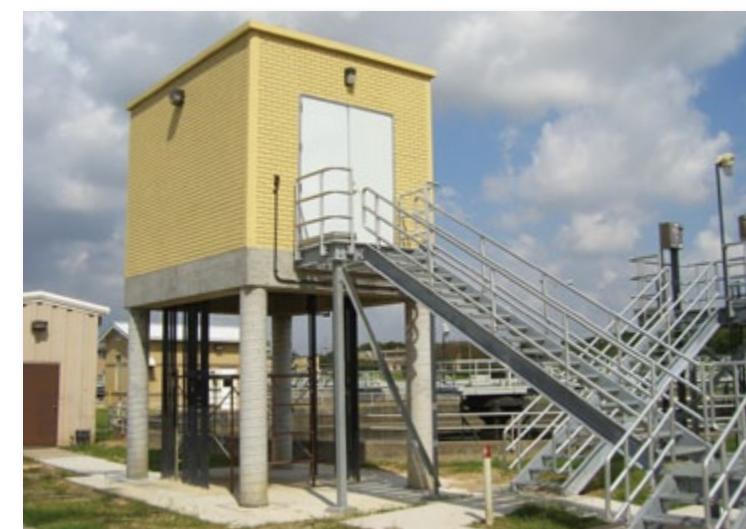
Wastewater Equipment Housing: Texas
