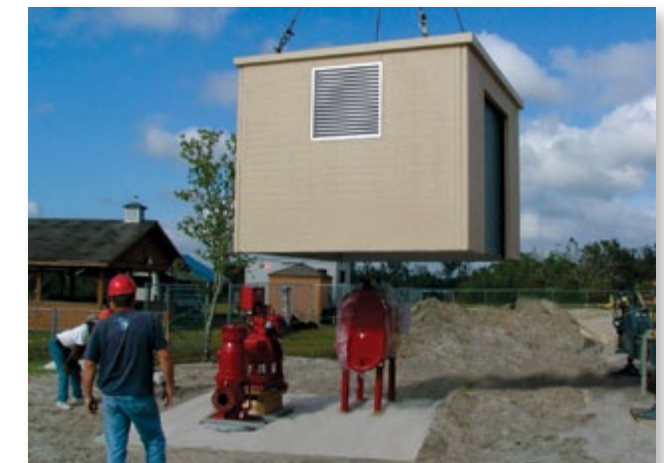
EASI-SET Buildings can also be delivered without a floor and placed on a pre-poured concrete slab.
