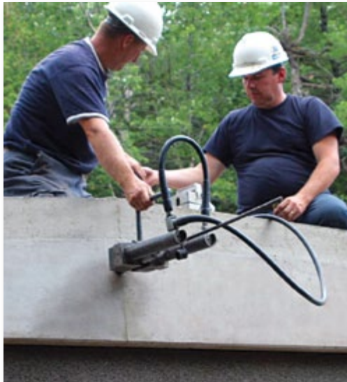
Post-tensioned roof for greater strength.
