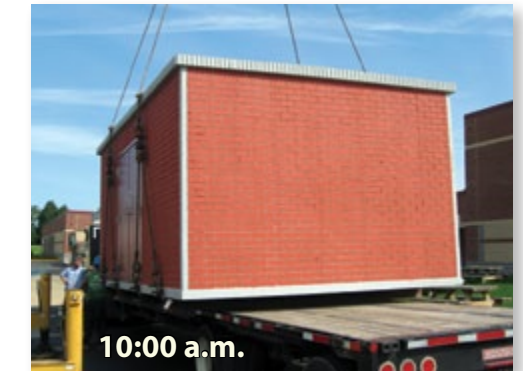
Delivered to-site completely pre-assembled, including precast concrete roof and floor.
