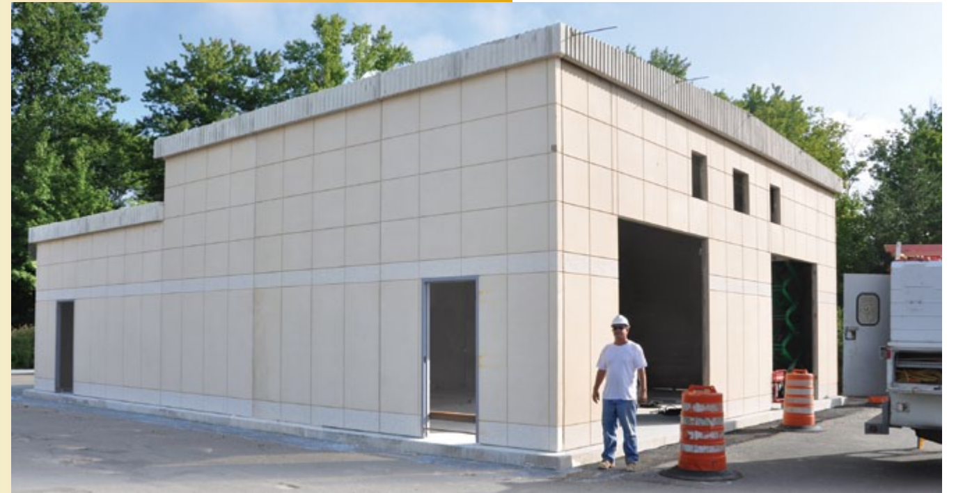
Vehicle Service Center: Virginia
