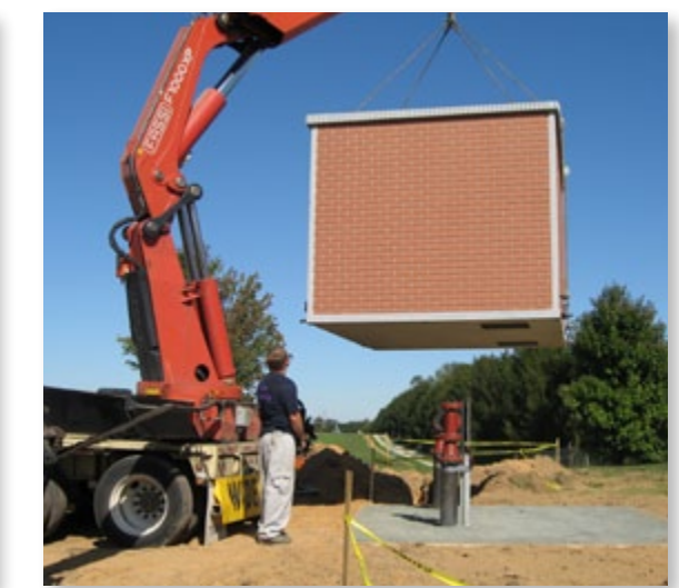
Well House, Virginia
