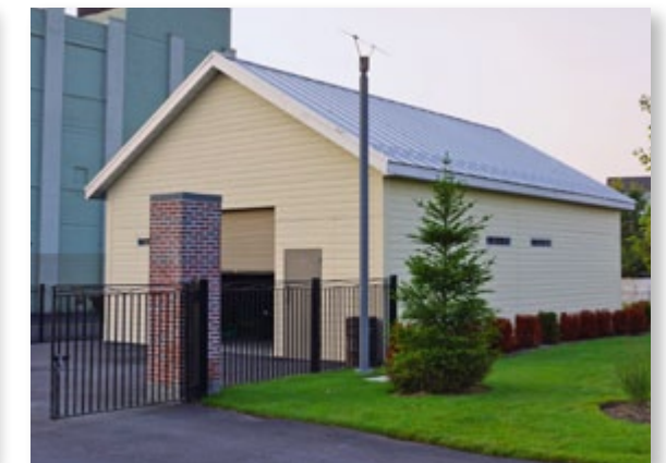
Maintenance Workshop: New Jersey
