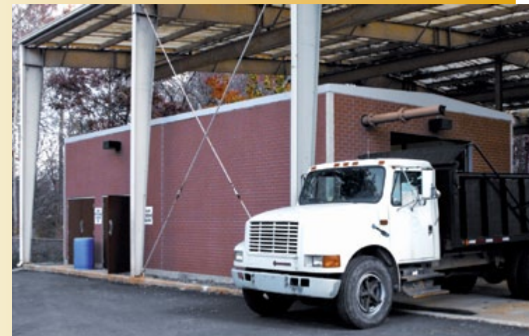
Solids Processing Plant: Virginia (installed within existing structure)
