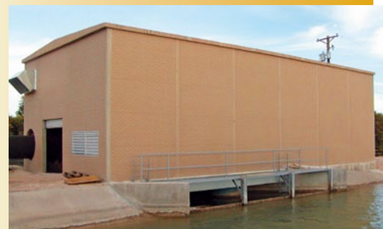
Water Treatment Pump Station: Nevada
