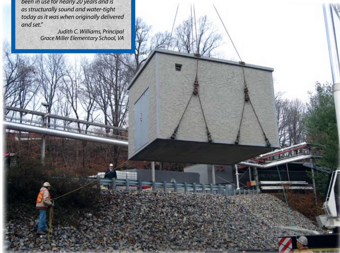
Easily installed at remote or restricted access locations: Connecticut
