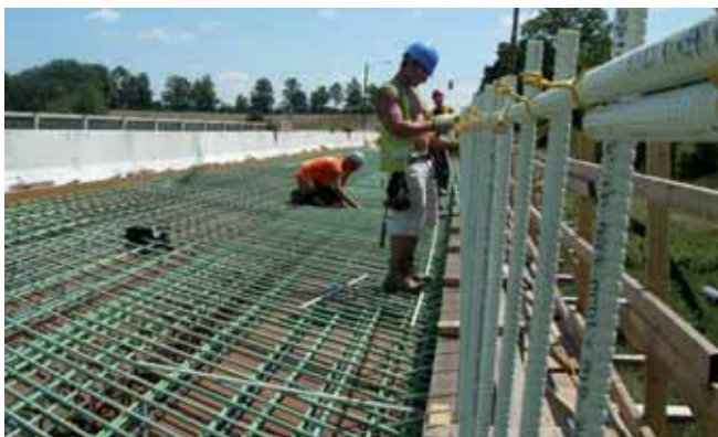
Irvine Creek Bridge near Fergus, Ontario, Canada
