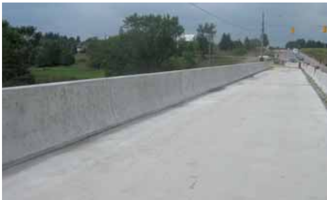
Irvine Creek Bridge near Fergus, Ontario, Canada
