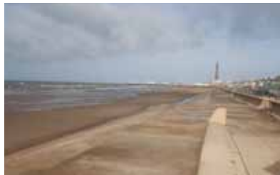
Coastal Defence, Blackpool (UK) Reinforcement of high quality aesthetic pre-cast concrete wall units for a seafront wall, instead of stainless steel. Owner: Blackpool Council Installation: 2007
