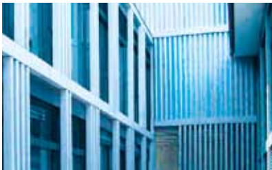
Facade of a school, Zug (CH) Extremely slim precast facade elements, corrosion prevention. Owner: City of Zug Installation: 2005 and 2006
